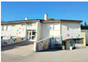
Primary school yard before works
