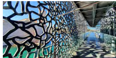
Mucem outer structure made with Ductal®
