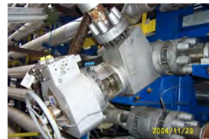
Rupture disc
